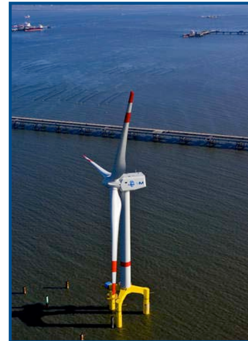
© BARD Engineering GmbH
